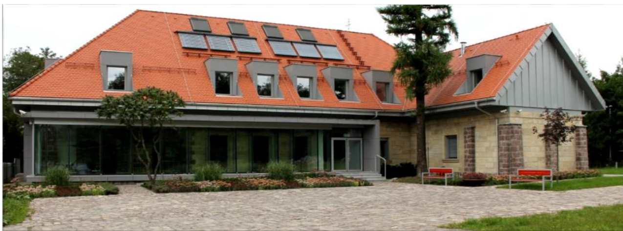
Figure 1. The main building of the Centre of Sustainable Development and Energy Savings of the Faculty of Geology, Geophysics and Environmental Protection of AGH University of Science and Technology in Miekinia, Poland
